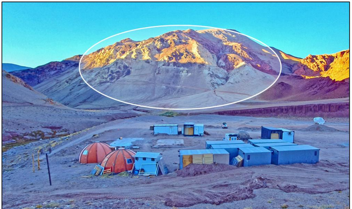
Figure 6. Picture taken from the TMT camp at 3300m altitude, looking south towards the Toro South target approximately 1km away. No new road work will be necessary, only the clearing of existing tracks.
