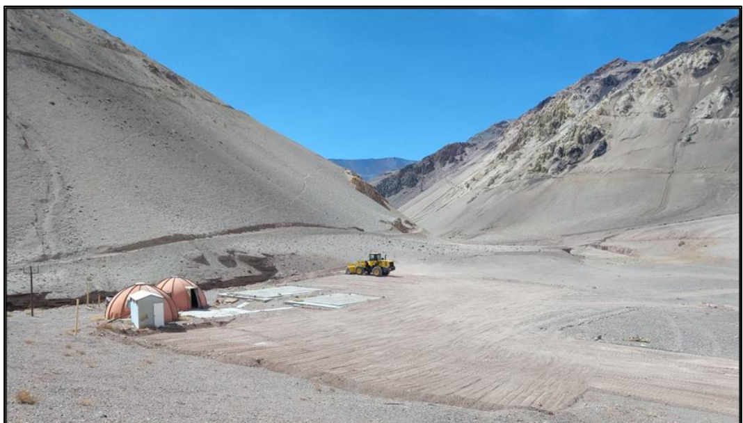
Figure 18: Toro Camp Groundwork Complete
