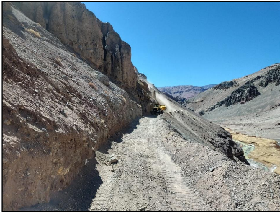
Figure 22: Internal track reinstatement at the Toro target
