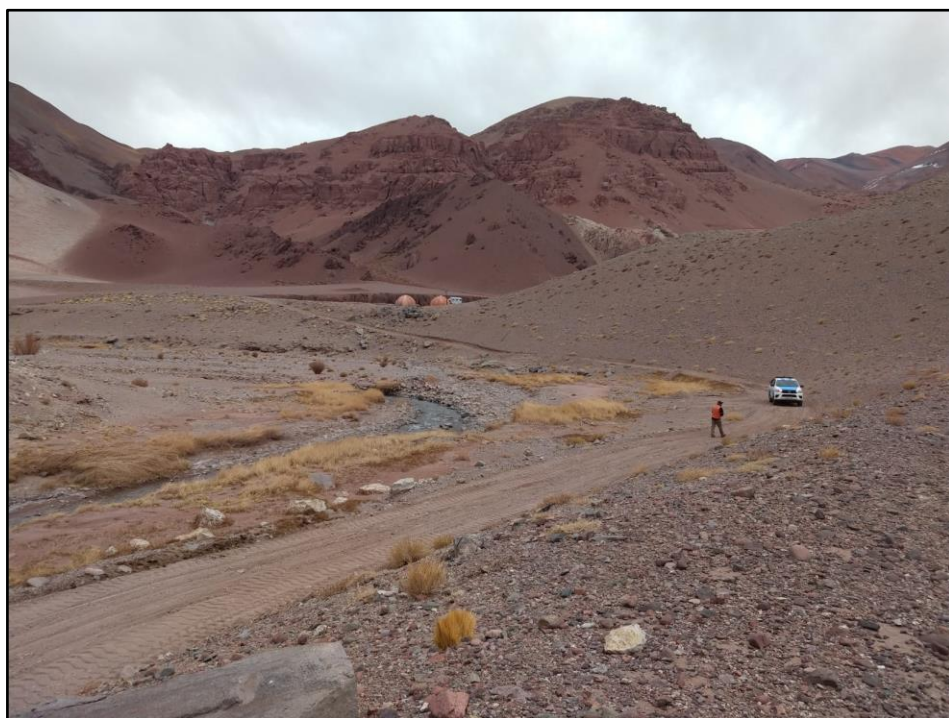
Figure 23: Access track reinstatement progressing north from the Toro Camp through the Toro tenement
