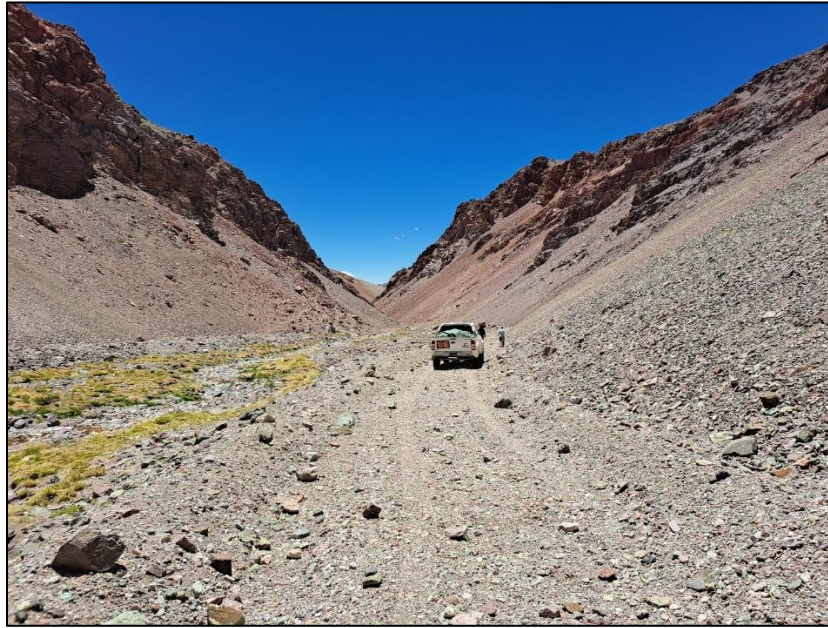
Figure 4: Access track in good condition that only needs minor maintenance
